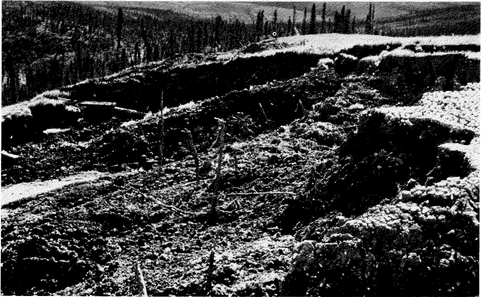
FIG. 7. Gulf Caribou N-25 wellsite, September 1975, following site restoration. Slumping and mass wasting occurred at the site of the initial leak of sump fluids. Photo: courtesy of W. Robson, Fisheries and Environment Canada, Whitehorse.
