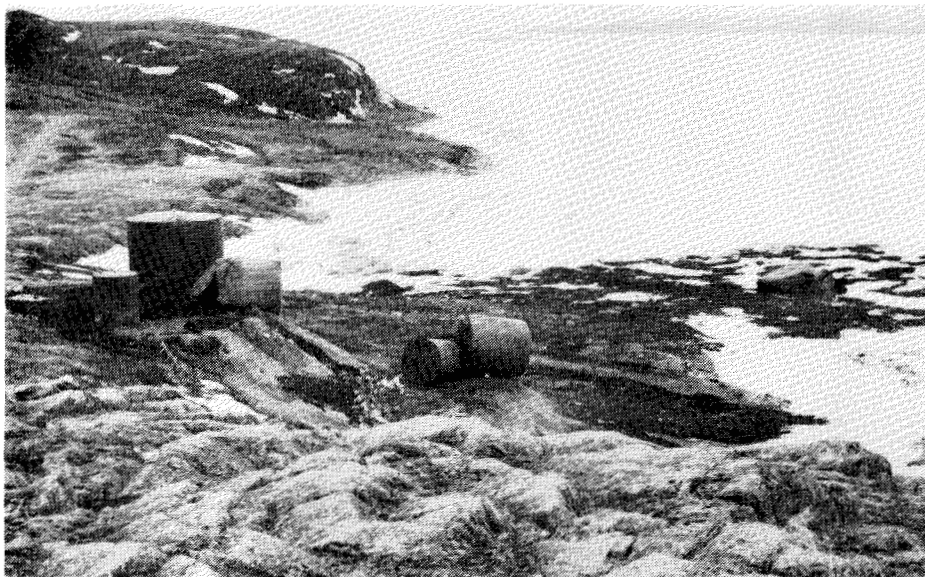
FIG. 1. A photograph of the spill site in which the 6 tanks in the tank farm may be seen. All of the tanks had been at the same level as the 3 on the left and all were damaged; however, the tank on the far left did not spill its contents of gasoline. The tank on the far right, well out on the foreshore, is understood to have been nearly empty at the time of the slide. View to the northwest at about higher high water on 18 June, about 10 days after the slide occurred, but before cleanup.
