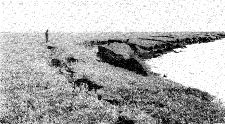
Fig. 2. Collapse of right bank through action of high waves generated by westerly winds.
