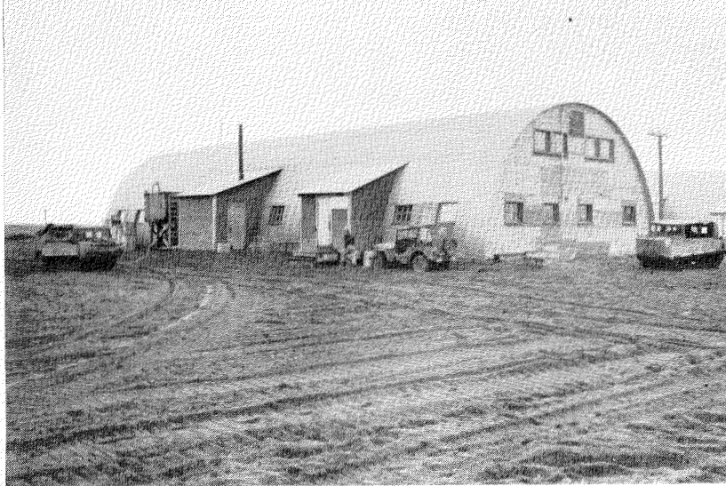
Newly modified two-storey laboratory building at Point Barrow photographed in July 1948.
